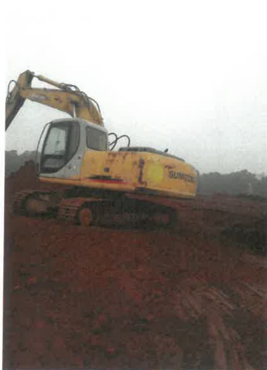
1#地块顺坡平整
