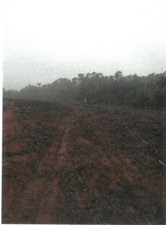
3#地块顺坡平整
